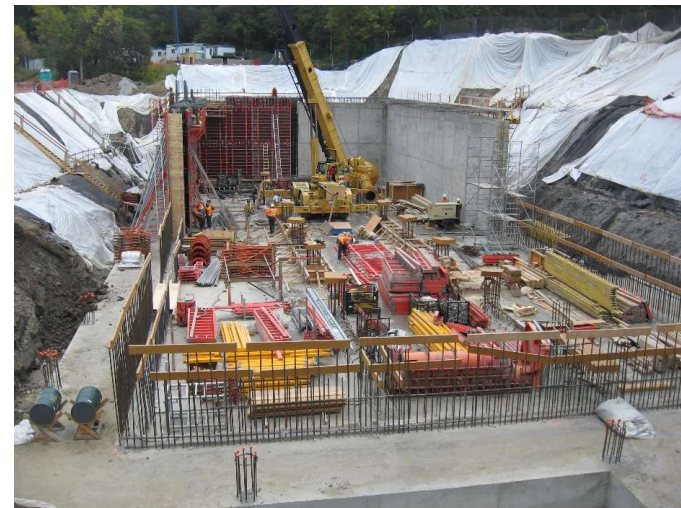
Example of tank excavation
